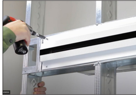
Screw through Mounting Flanges to Framing
