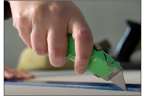
Cut Drywall to Cover Mounting Flanges
