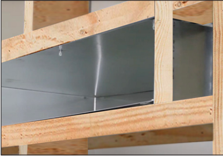
Install Ducting within Wood or Metal Framing
